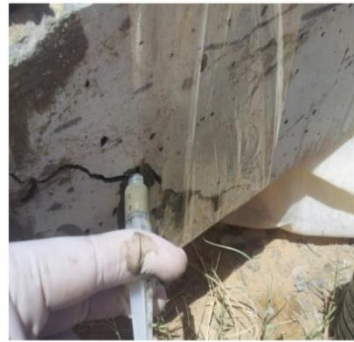
Beam during repairing using the injection technique.
