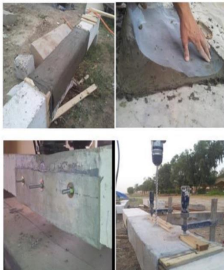
Figure 10. Strengthening using Ferrocement [17]
