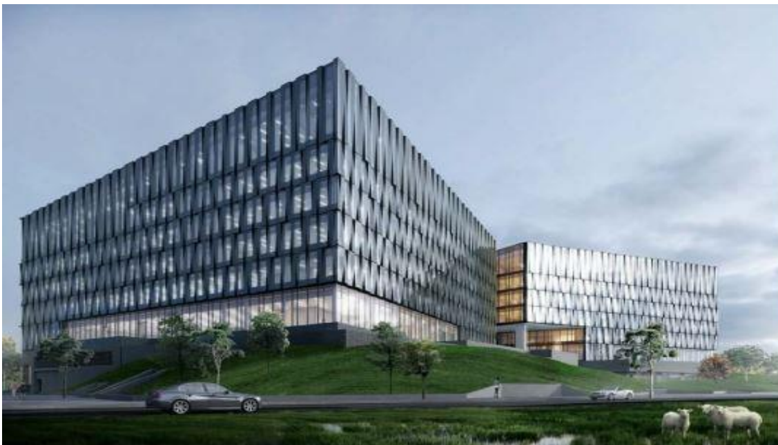
Figure 5. Nordea Bank Headquarters: south-west view. [Source: Henning Larsen Architects]
