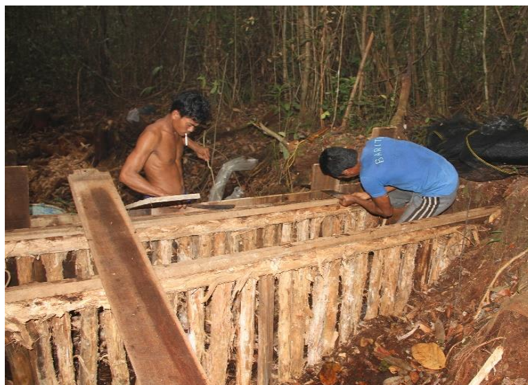
Figure 2. Construction of canal barriers in tropical peat swamp forests
