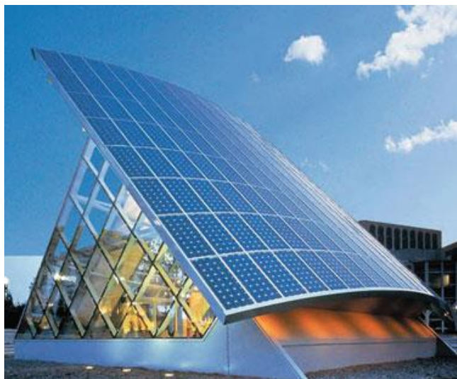
Figure 7. PVs integrated on a curved roof, BP solar showcase in Birmingham [26]
