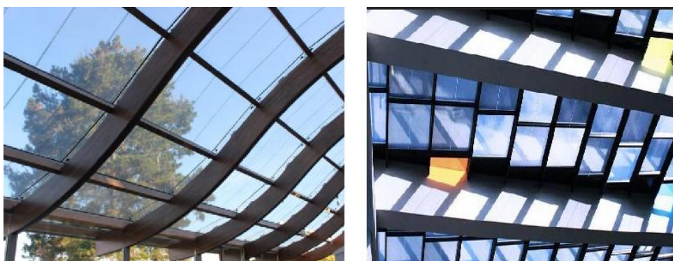
Figure 6. BIPV slide-like shape glass in the form of skylight OnyxSolar [26]
