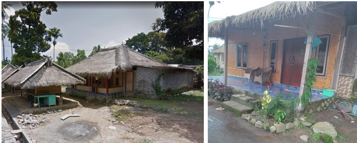
Figure 13. Bale Mangina which has undergone modern material modifications (Source: Google Earth, 2016; informant documentation, 2025)
