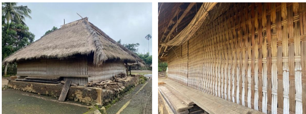
Figure 9. Bale Mangina walls still use split bamboo woven material (Source: researcher documentation, 2025)
