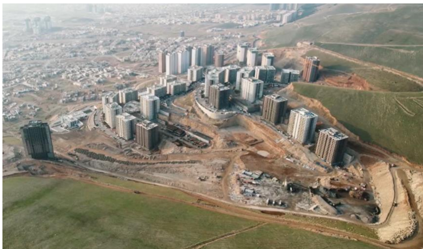
Figure 7. Cutting the mountainous area and building a residential complex
